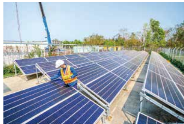
The Group’s large-scale residential project in Shap Sz Heung became the first construction site in Hong Kong to install solar panels to generate renewable energy for on-site offices.
